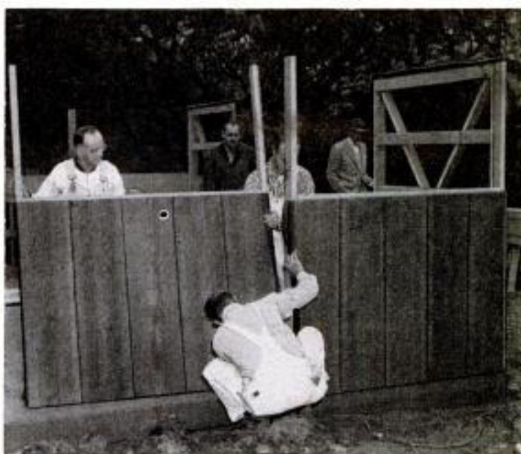
Adjoining studs at ends of panels form post to support roof. Below, home made of same panels as model has different look
